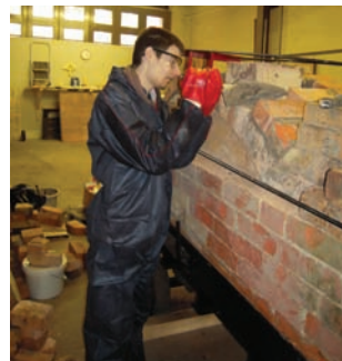
Brandon working on the furnace
