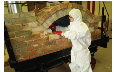
Becky also working on the furnace
